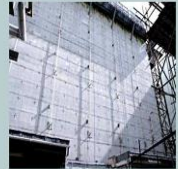
Pile Fuel Cladding Silo
