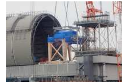
Crane for installing fuel handling equipment
