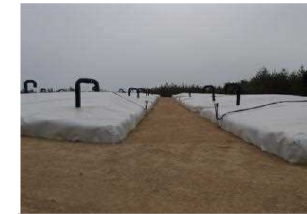
Temporary trimmed trees storage pool
