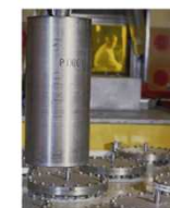
Bolted wellheads containing fuels, handled via a control room © CEA-JOLY
