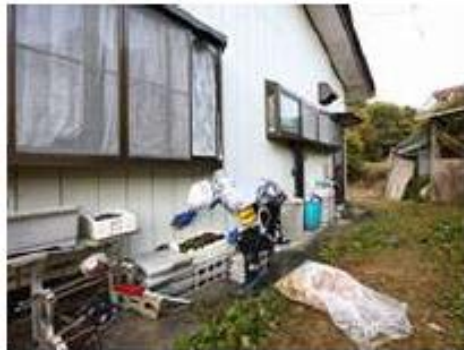
2 oct House wall: wiping
