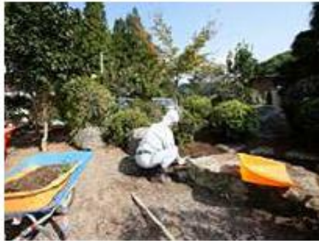
House garden: removal of topsoil
