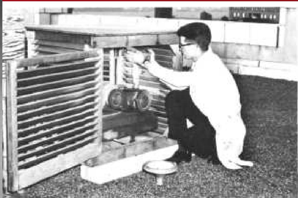
*Radioactive fission-product concentrations in ground-level air are measured at 50 stations at the same longitude, at intervals from Greenland to the southern tip of South America. From these measurements the mixing of fission debris in the atmosphere at different latitudes is studied. This photo shows a sampler on the roof of the AEC's Health and Safety Laboratory in New York City. This sampler filters dust from 10,000 cubic meters of air each week.*
