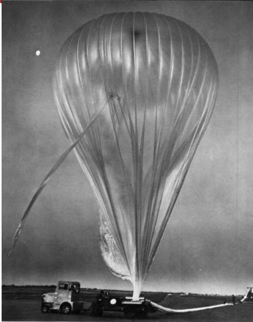
*This high-altitude balloon is being prepared for launching at Goodfellow Air Force Base in Texas. The balloon carries air-filtering devices to collect atmospheric particulate samples, which are analyzed for various radionuclides. This information is useful in interpreting movement of radioactive debris from its point of injection into the atmosphere to its deposition on the earth's surface.*
