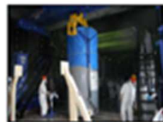
① Installation of cesium adsorption tower
