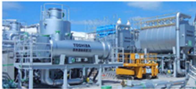
Evaporative concentration apparatus (3A, 3B, 3C)
