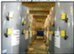
② Cesium adsorption towers
