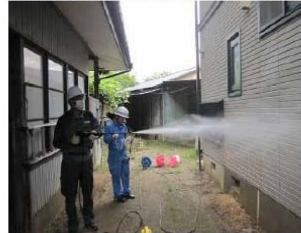
Wash wall with high-pressure water
