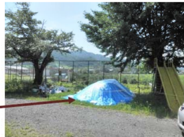
Temporary storage of removed soil
