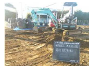
Excavation of the surface soil
