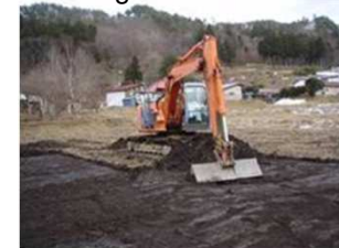
Vertical replacement of soil
