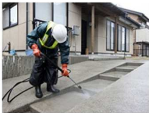
High-pressure cleaning
